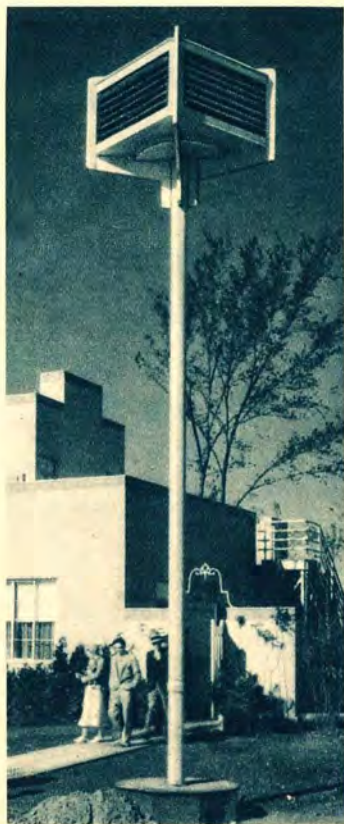
One of the 114 loud speakers in the World's Fair public address system
