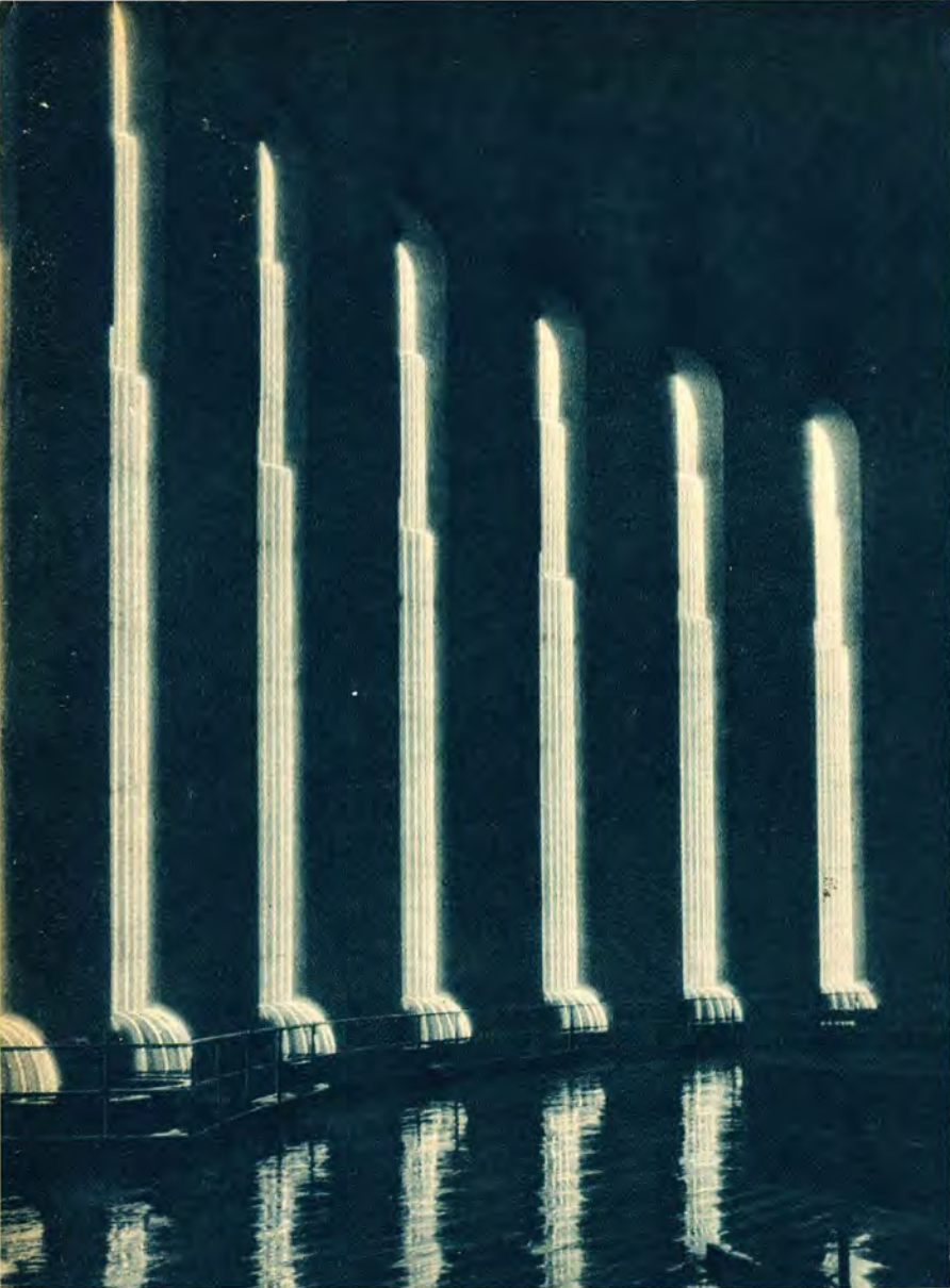
A rainy night at the World's Fair, showing the graceful and symmetrical cascades that ornament the semi-circular facade of the Electrical Building. The effect is striking and modernistic, in keeping with the spirit of the Century of Progress Exposition
