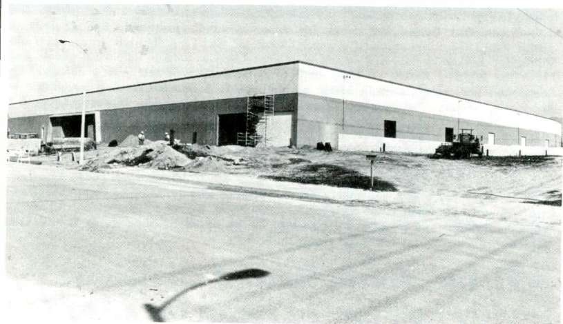
New A&M Sun Valley central warehousing facility.
