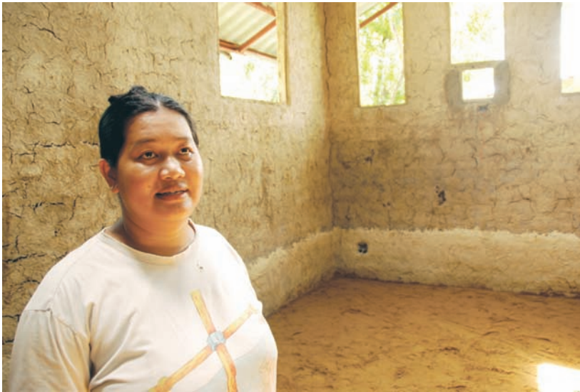
Pairin Pongsura, Manager of Siambaandin Co., Ltd., stands inside a mud house under construction. The venture has as its goal environmental conservation.
