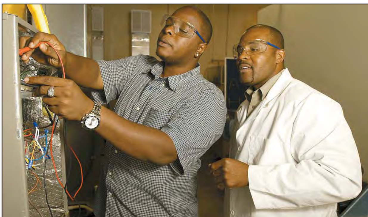
Henry Wehner (left), practices along with Fred Loving, lead instructor the of air conditioning, heat and refrigerator department at the Cabarrus Business and Technology Center in Charlotte, N.C.
