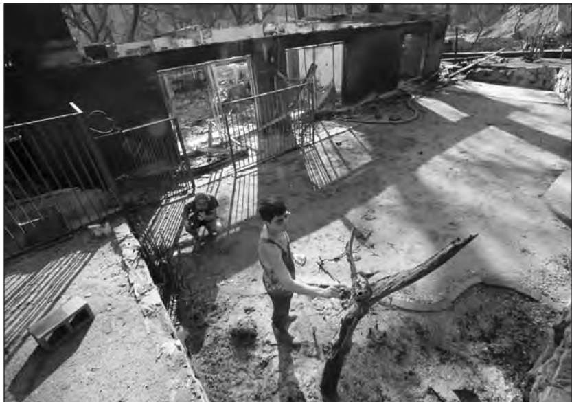
Niko Solario , an artist who had lived in his friend's home on Stonyvale Road off and on for five years, prepares to videotape the ruins of the home after the Station fire swept through Big Tujunga Canyon in the Angeles National Forest, just outside the Sunland area of Los Angeles.
