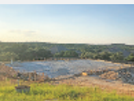
House foundation laid in Dripping Springs ETJ MAGGIE Q. THOMPSON
