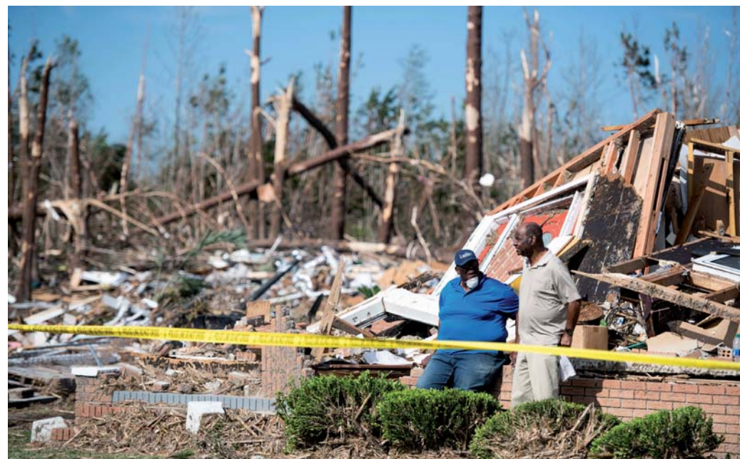
Two men talk in front of a destroyed home in Nixville, South Carolina, on Monday.
