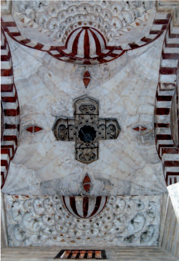
13. Vestibule of the mosque of Sultan al-Mu'ayyad (1421).
