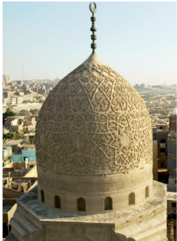
12. The mausoleum dome of Sultan Qaytbay (1473) (photo Bernard O'Kane).
