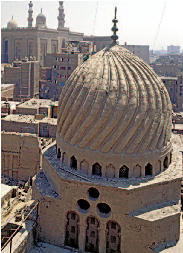
11. The mausoleum dome of the emir Uljay al-Yusufi (1373) (photo Bernard O'Kane).
