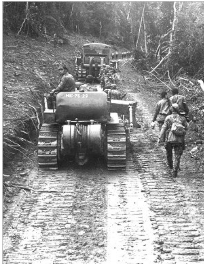
Figure 4.5: Bulldozers Used to Build Military Road in Eastern Angola
