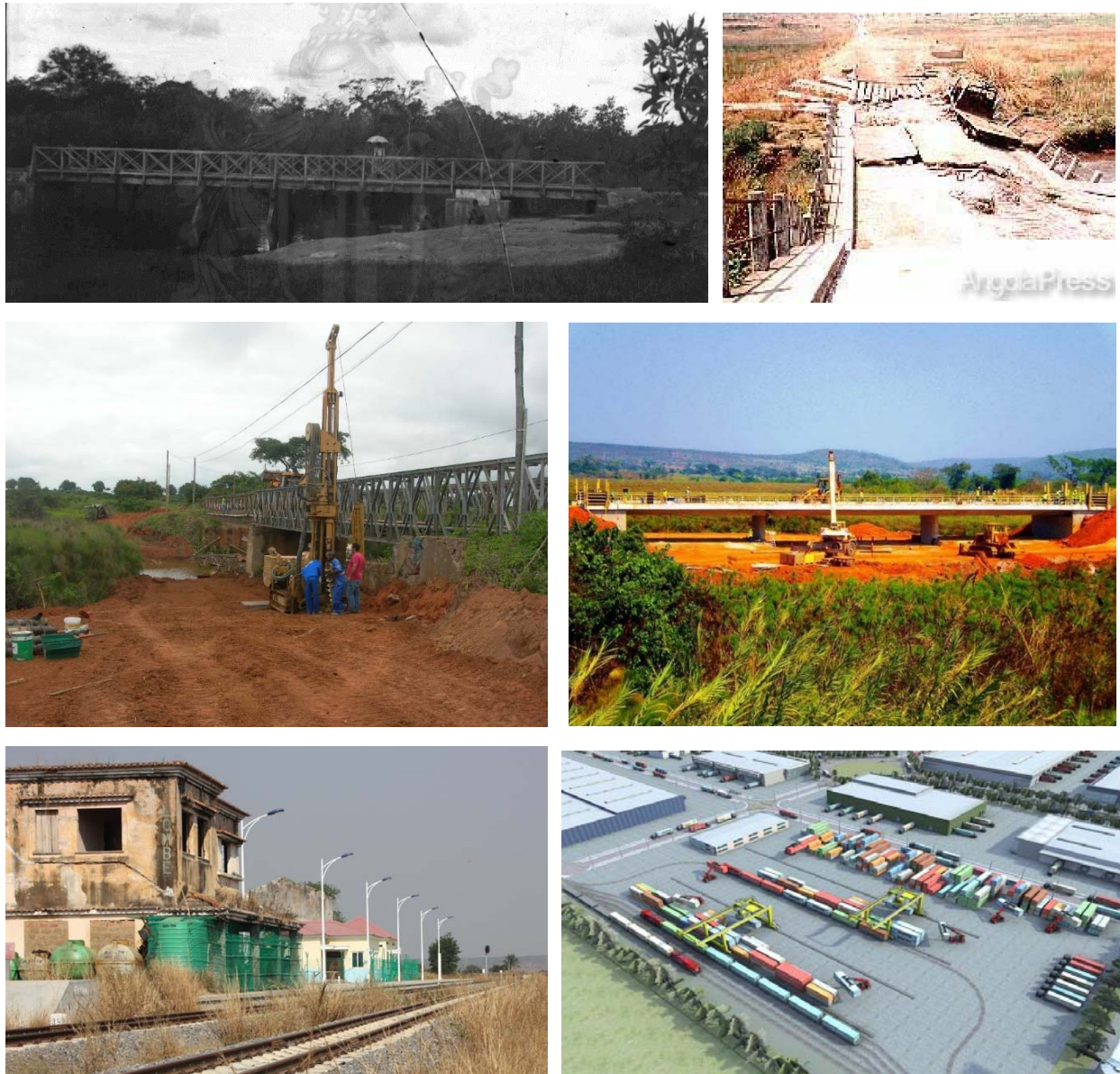
Figure 4.2: Lombe Road and Rail Bridges and Infrastructure, 1907, 2008, and 2013
