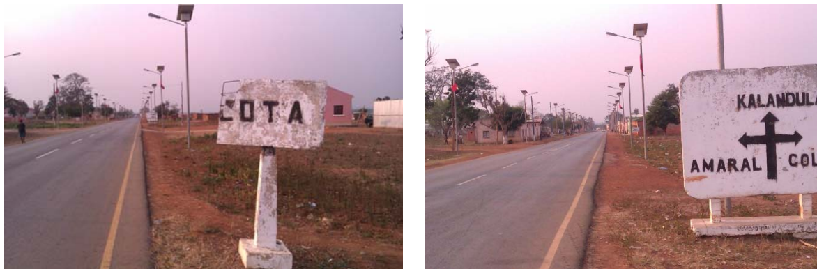
Figure 1.4: Road through Kota
