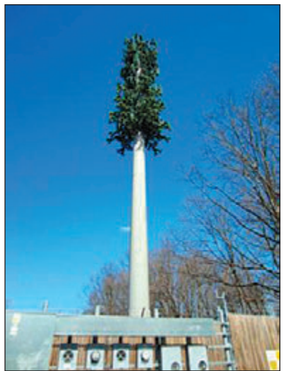
One version of the so-called "monopine" cell tower disguise. AT&T had said disguising the tower might be one option but neighbors said the 'tree' would be 90 feet taller than the area's tree line.
