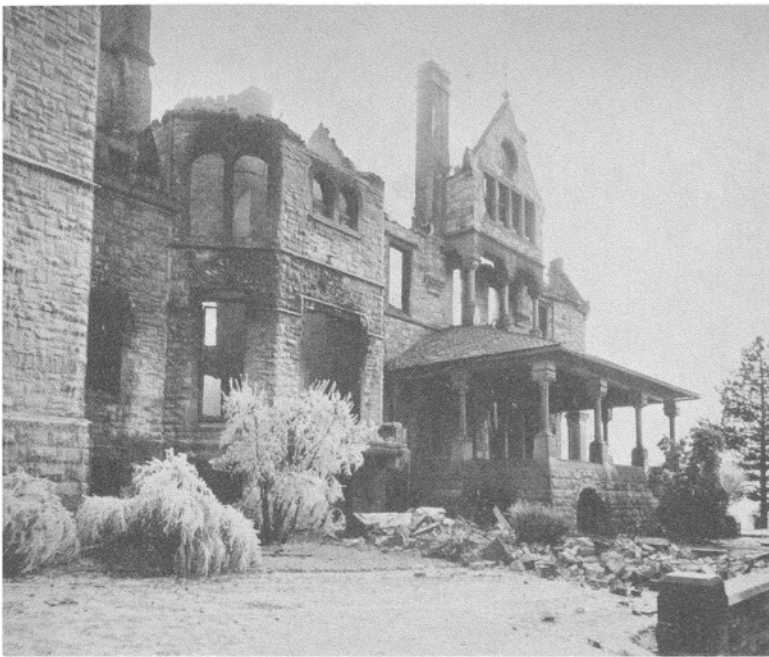
Gutted remains stand without roof, beyond saving.
