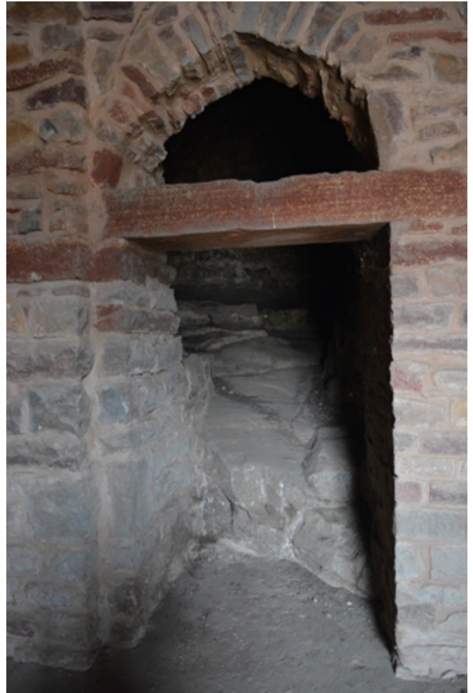
Fig. 1. Cell at the base of the Jami Mosque.
