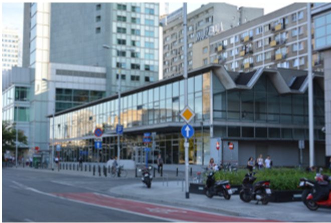
Fig. 3. “Emilia” pavilion, where the Museum of Modern Art in Warsaw was operating in 2012-2016 (afterwards it was dismantled). It is surrounded by socialist residential blocks and modern office buildings. Opposite, across the street, is the Palace of Culture and Science. (Figs. 3-6 © Author).
