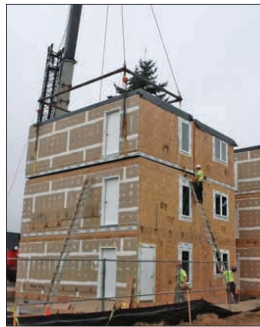
Construction workers oversee the stacking of pre-fabricated modules into the Kah San Chako Haws apartment building in Southeast Portland. The nine-unit development is an experiment in quicker and cheaper construction of low-income housing.
