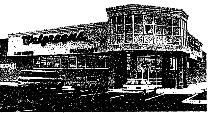
Pointe Plaza, a new 335,000-square-foot shopping center by Tucker Development Corporation (TDC), recently opened its first store, a 14,000-square-foot Walgreens, on Saturday November 27, 1999. Located at the northwest corner of Touhy and Central Avenue, other anchor tenants include a 133,000 square foot Wal-Mart, 58,000 square foot Cub Foods, 97,000 square foot Babies R Us, and a 30,000 square foot Office Depot. Additional tenants include Blockbuster Video, Starbucks, Wolf Camera and Bennigan's. With remaining retail space still available, additional leases are expected to be signed soon. Grand opening is scheduled for Spring 2000.
